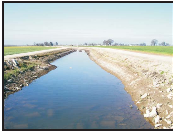
Laguna Irrigation Canal
