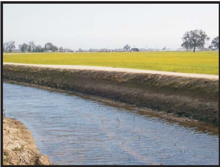
Laguna Irrigation Canal
