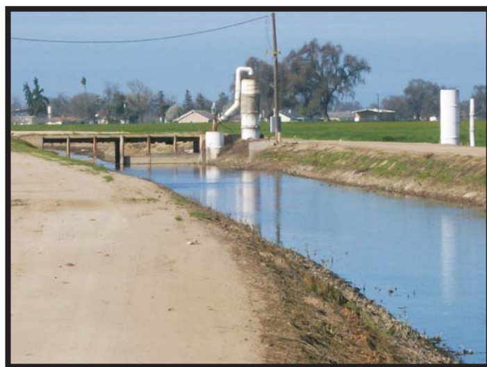
Laguna Irrigation Canal and lift pump
